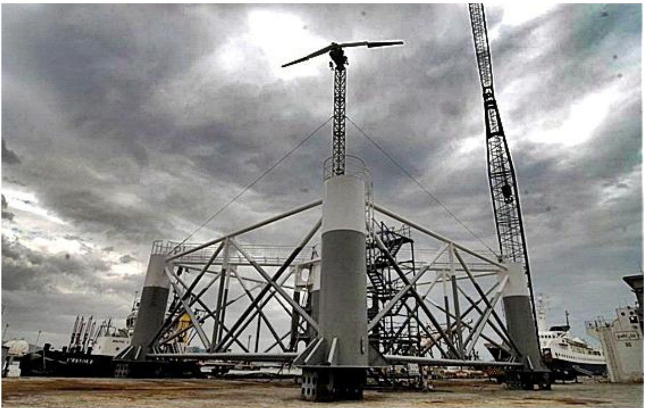
This photo is of the Hydrhada experimental wind turbine for desalination being trialled in the Aegean Sea, Greek Islands
